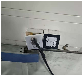
TAIPAQ Plant baking station socket damage before/after improvement
