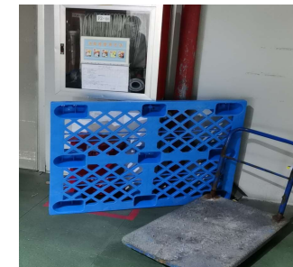
TAIPAQ Plant fire facility blocking before/after improvement
